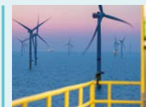
In collaboration with Hitachi Energy - early works agreement for TeneT's 2GW offshore wind programme
