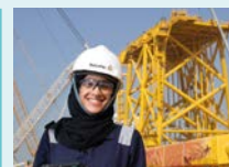
Design, build and install of two HVAC platforms for Hollandse Kust Zuid
