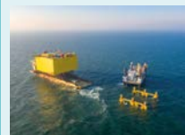
BorWin3 jacket and topside installed via mammoth floatover
